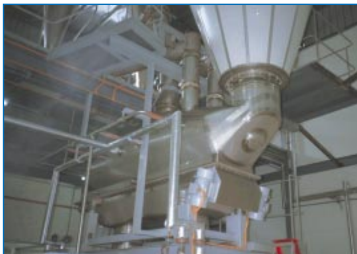
Figure 5. Conical section of a large spray dryer with secondary fluid bed dryer
